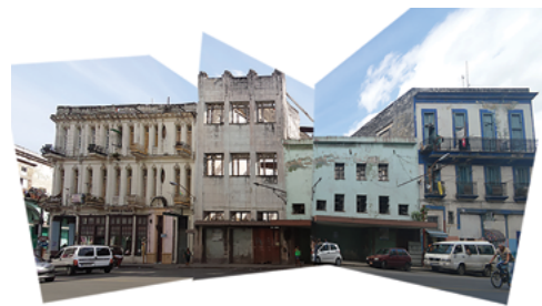
FACADE AVANT INTERVENTION
